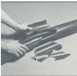
Remove damaged or faulty ducting
